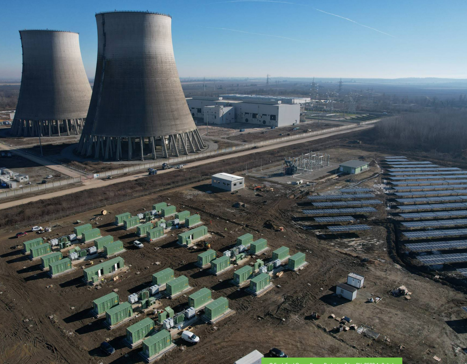
© Enel, Enel Green Power Projects - Trino PV+BESS 1+2, Italy
