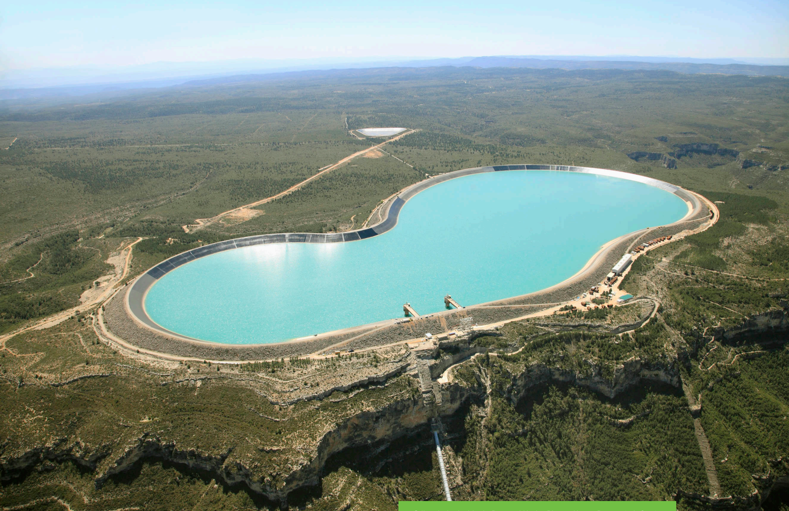
© Iberdrola, La Muela Pumped Hydro Plant – Upper Reservoir 1, Spain
