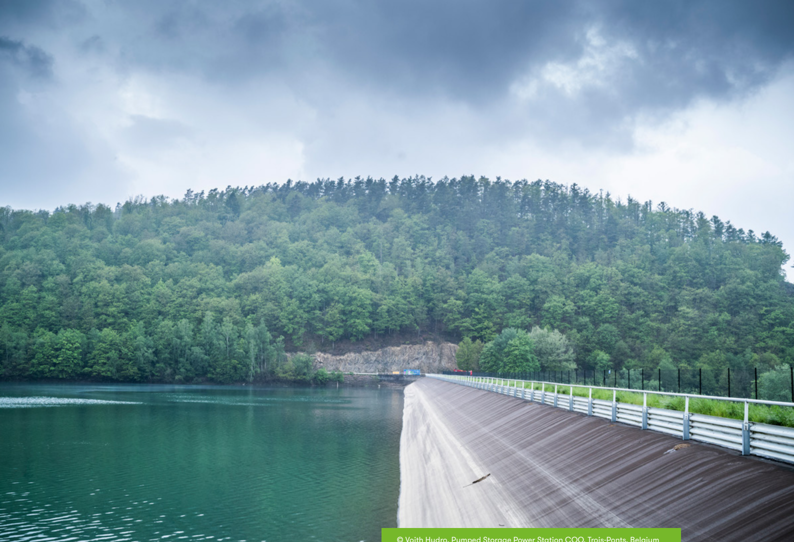
© Voith Hydro, Pumped Storage Power Station COO, Trois-Ponts, Belgium
