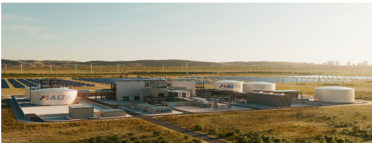
100MWe synchronous pumped heat electricity storage system to replace gas fired grid power © Malta
