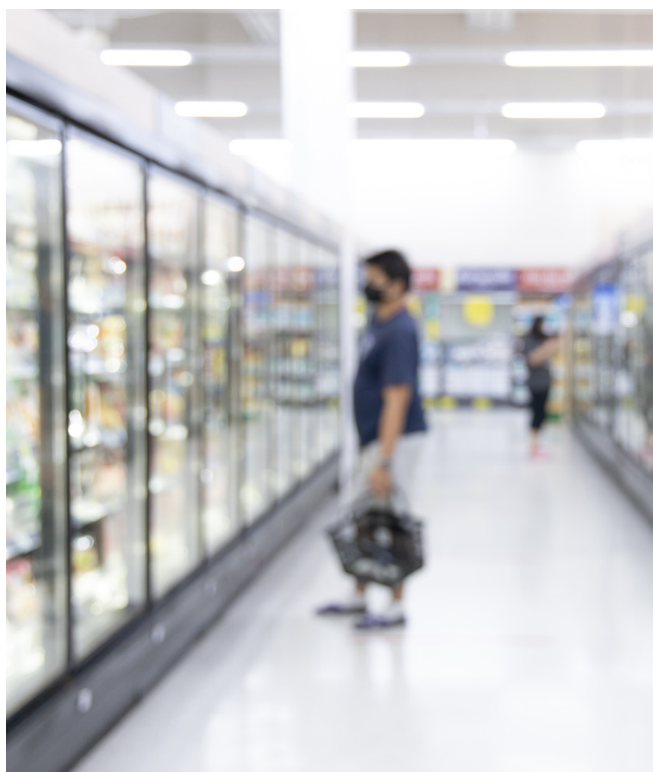
Refrigeration aisle in supermarket
