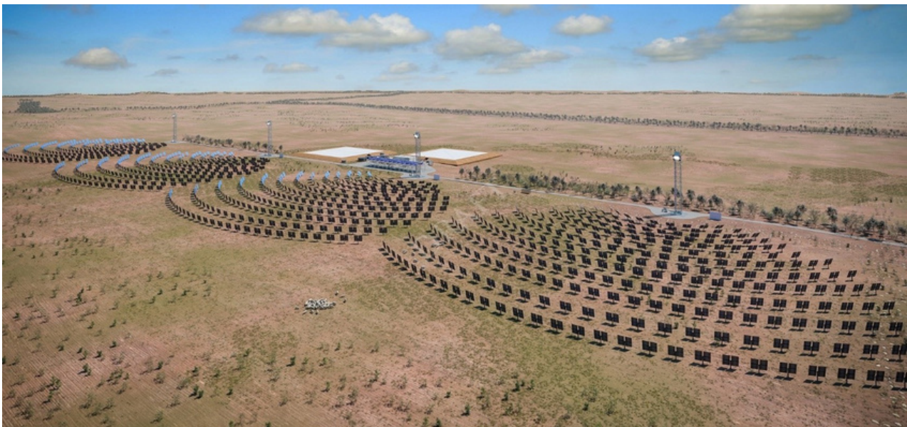
Project at Carwarp, Australia with 4MWp of solar + 3MW of AC power from the heat engine connected to 50 MWh of thermal storage © SLB
