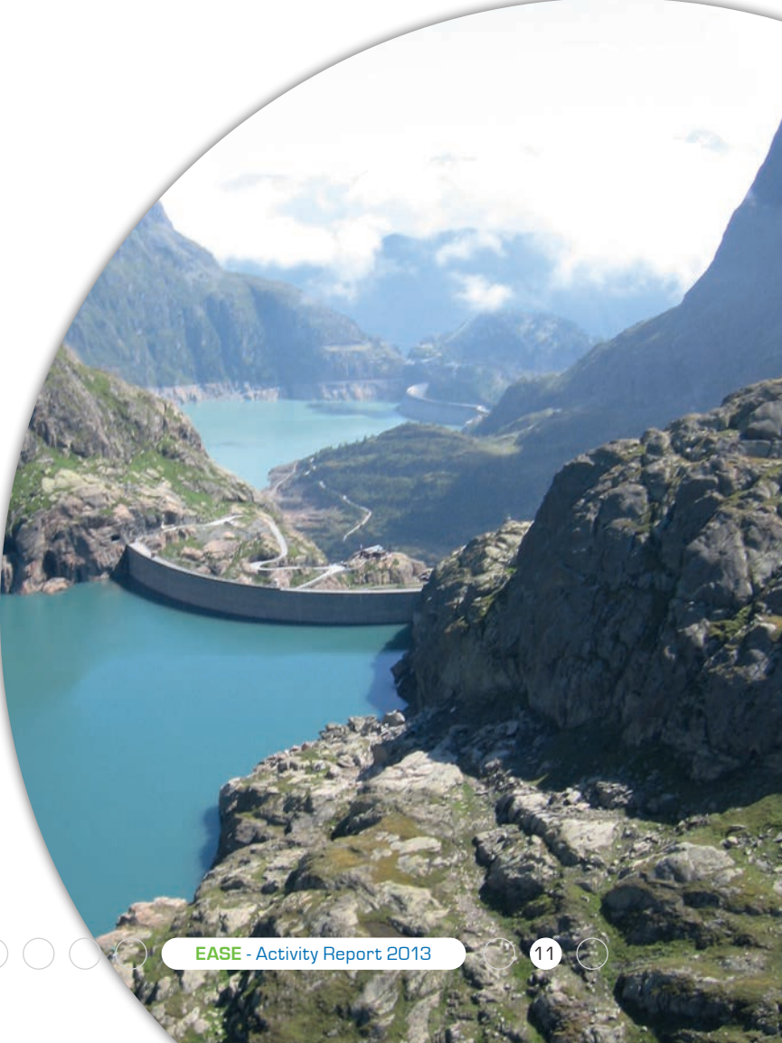
Variable Speed Pumped Hydro Storage power plant Alstom
