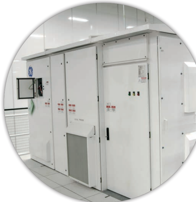
Inverter GE Energy Storage
