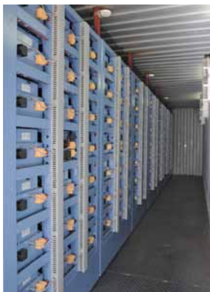
TDK, Battery Modules in racks
