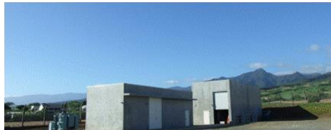
NA S Battery Energy Storage → Ensure production
