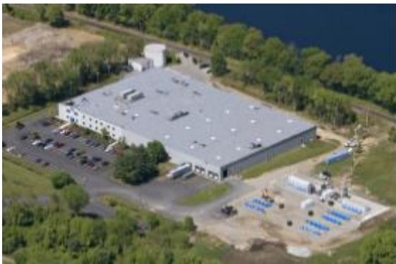
Tyngsboro, MA 0.5 MW Operating since 2008
